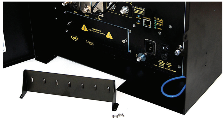
Figure 4-9: Cable Management Bar Removed
